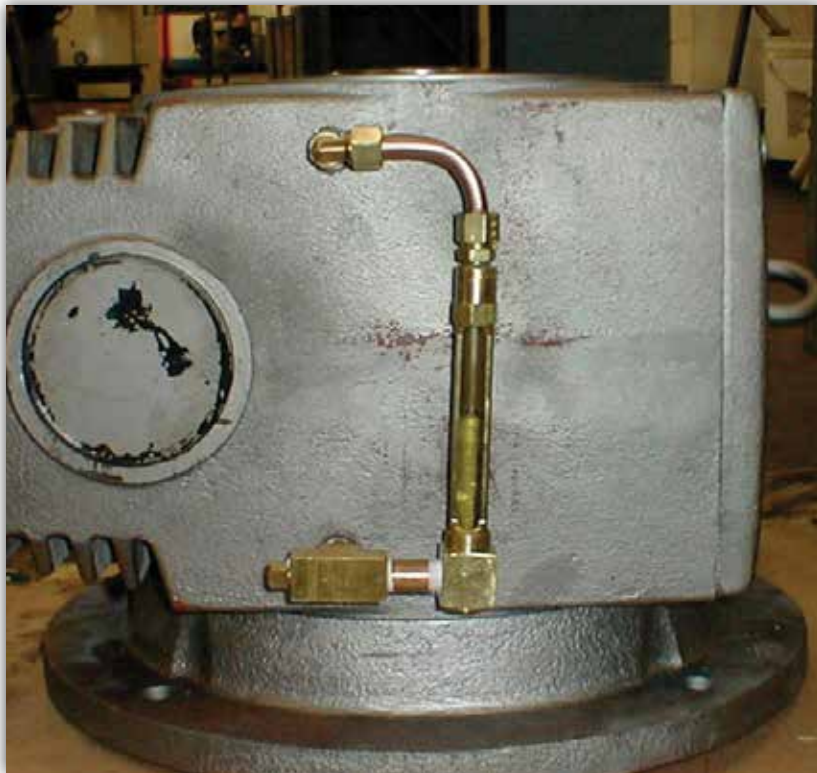
Closed system liquid level gauge with pressure balancing line connected to a gearbox housing
