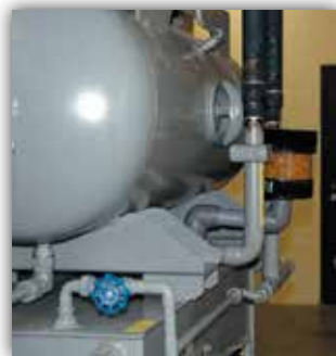
Watchdog Breather installed on a hydraulic reservoir
